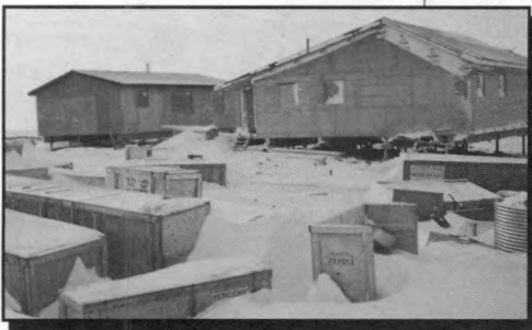
Homeownership Assistance Program (HAP) unit under construction, Repulse Bay
