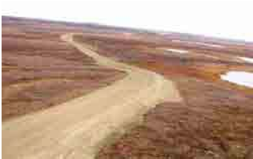
Photo 5.2-3 Partially complete access road from Tuktoyaktuk to Source 177
